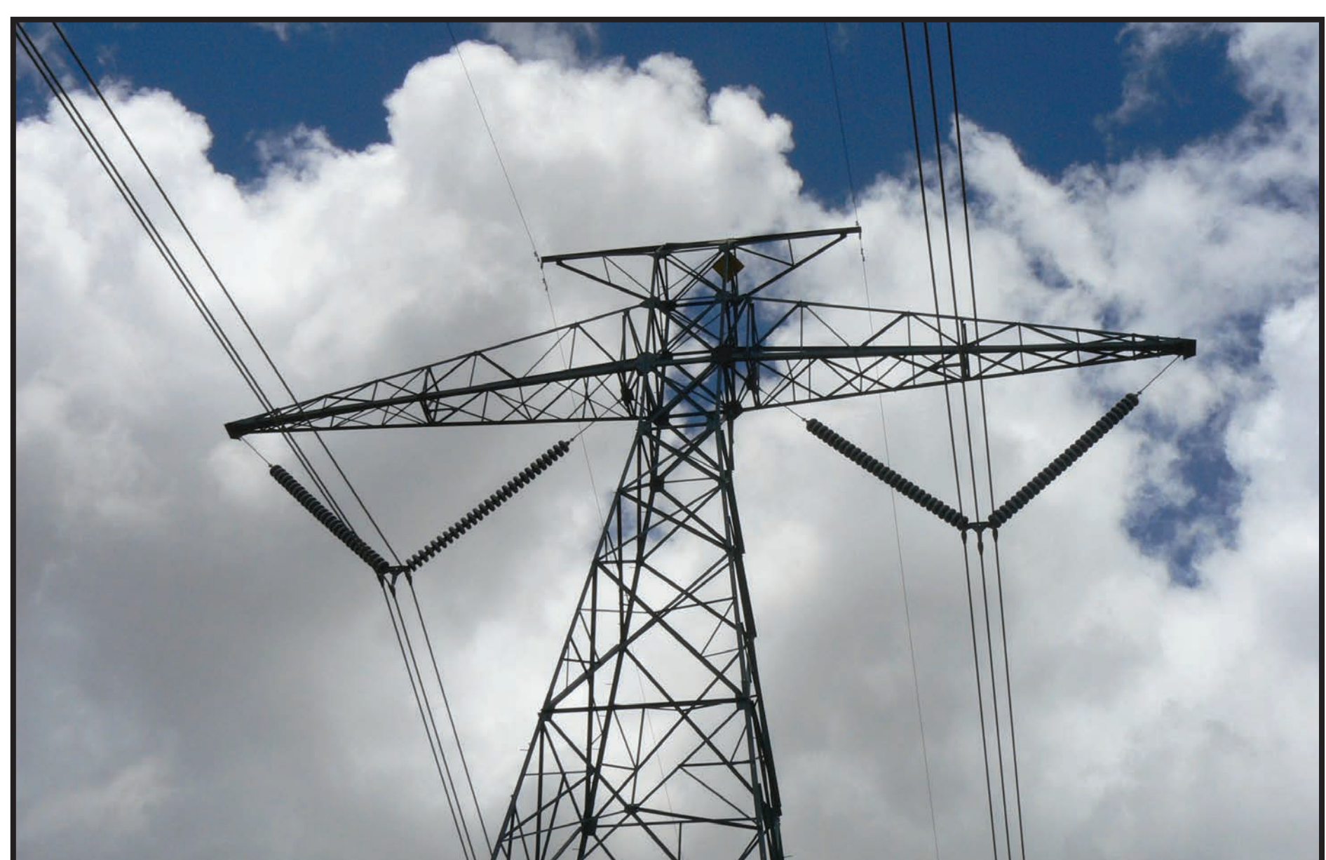
Representative photo of self-supporting lattice tangent structure.
