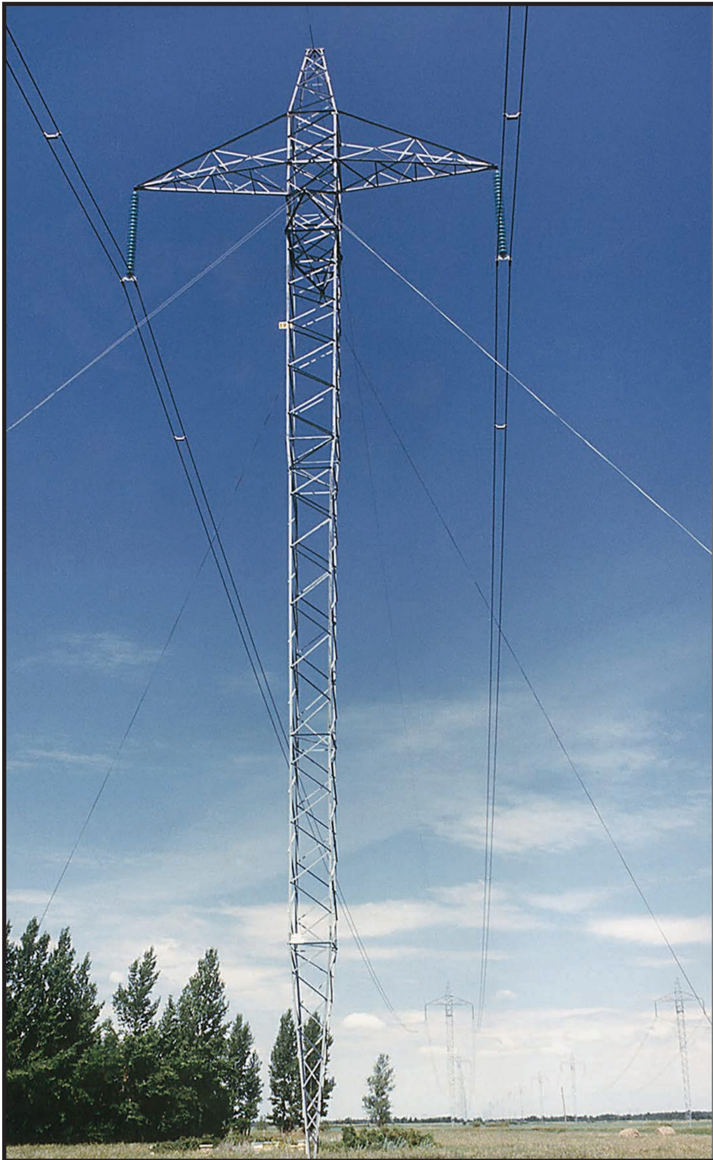
Representative photo of guyed I-string lattice tangent structure.
